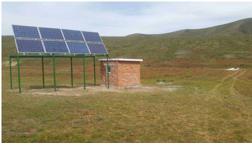
Solar panel array to power a pump that provides water to an artificial water hole for Asian wild horses. Photo by Usukhjargal Dorj
